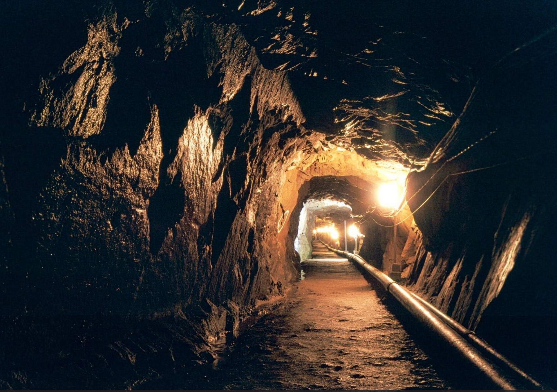
Le 3 eme Tunnel
