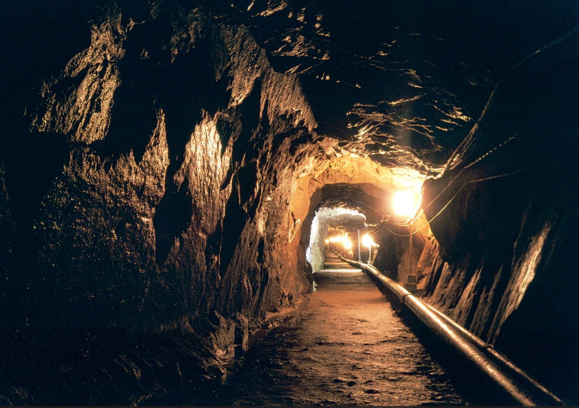
The 3 rd Tunnel
