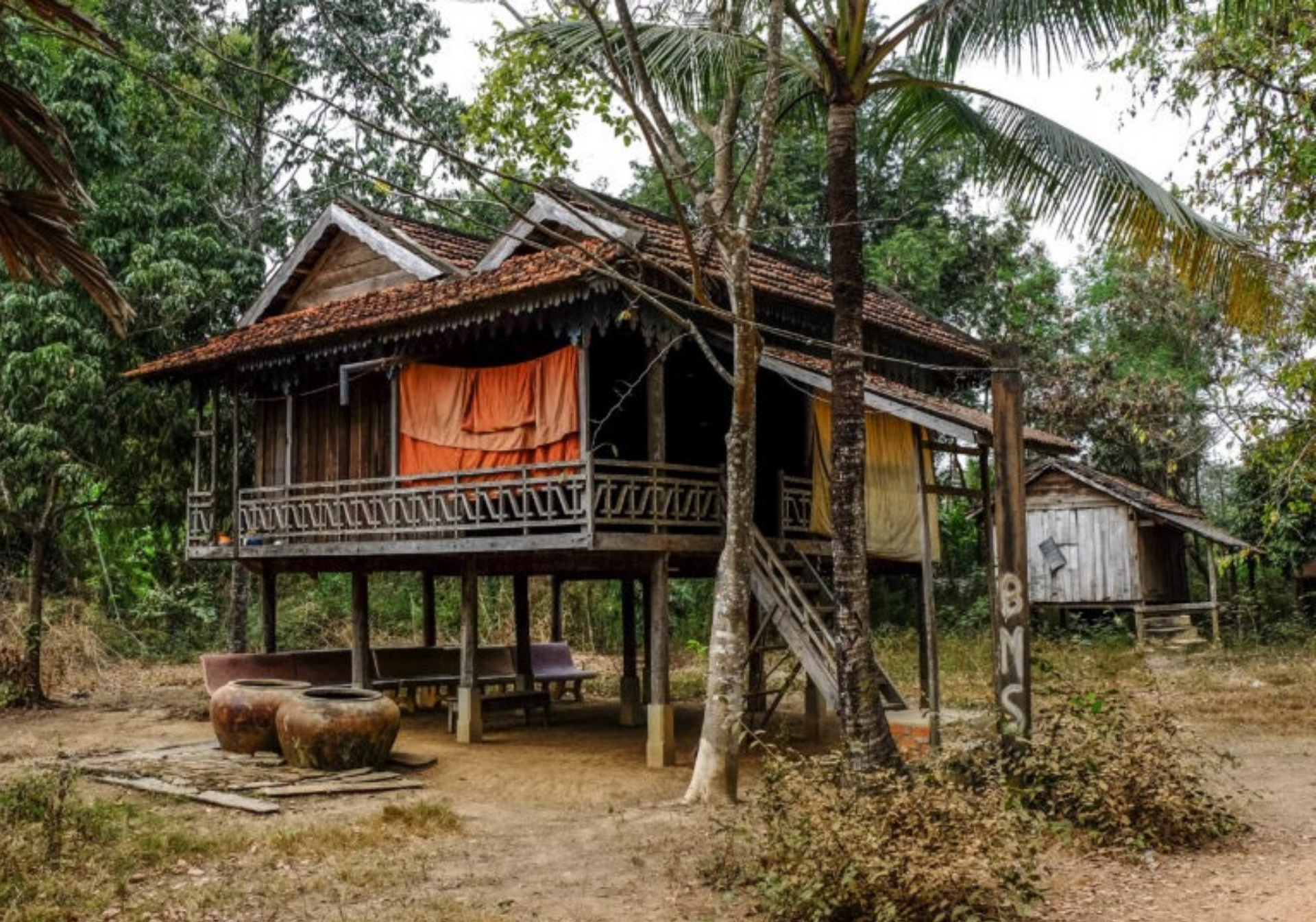
Siem Reap – A House on Stilts
